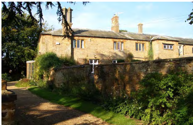
The converted former stable block and coach house to Great Billing hall, listed grade II, are of historic significance as surviving buildings associated with the Hall
