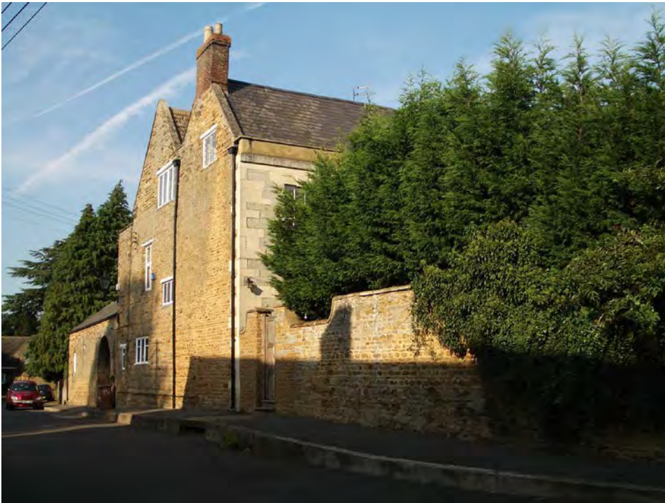
The Old Rectory on Elwes Way – 17 th century coursed limestone re-faced with smooth ashlar blocks in the 18 th century; limestone was normally used in coursed rubble form and cut ashlar is not common within the village
