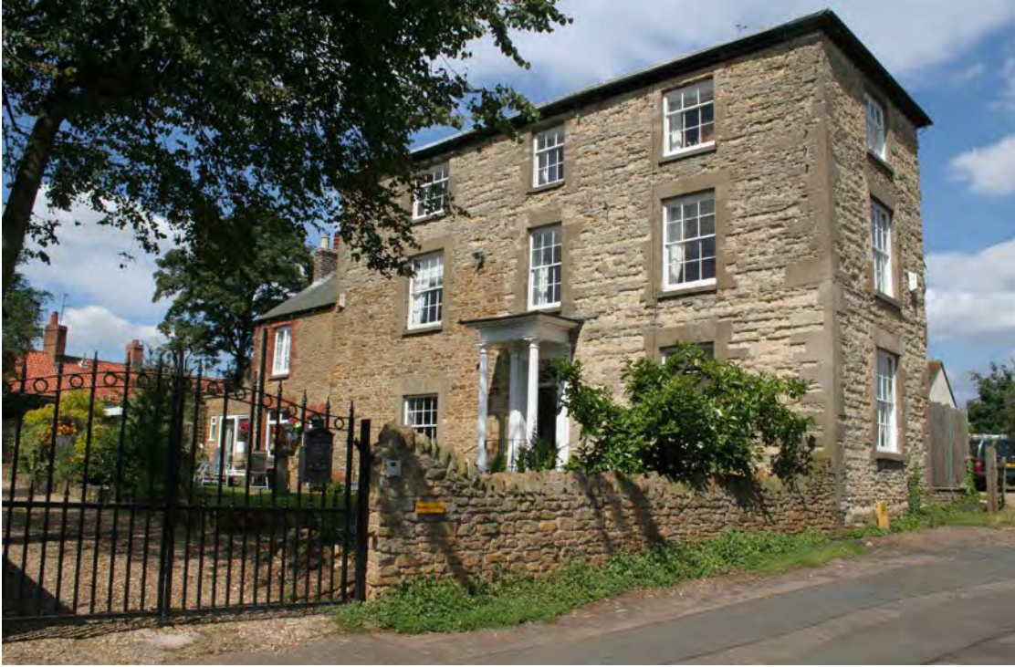
This Georgian house on Cattle Hill is urban in character and reflects the diversity of building styles within the village; coursed limestone with more durable flush quoins and hipped slate roof. The Doric style porch and tall sash windows are attractive Classical features of late 18 th & early 19 th century buildings.
